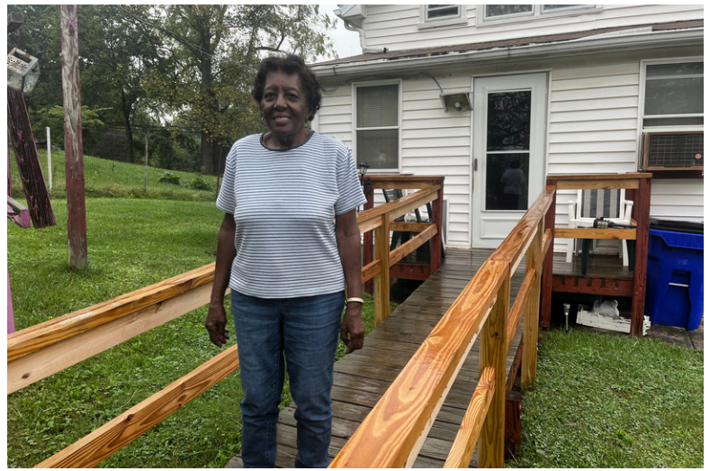
Catherine Biggus standing proudly on her repaired ramp.
